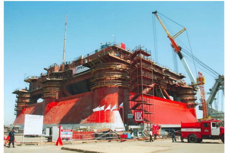
Construction of an offshore platform for Yu. Korchagin field development.
