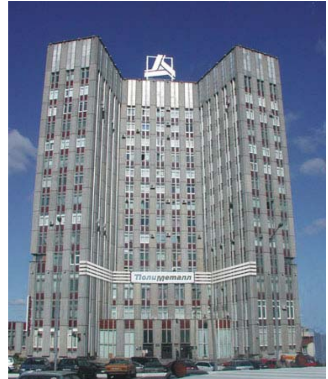
Headquarters in Saint-Petersburg
