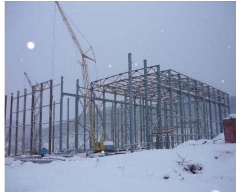
Flotation concentrator in construction
