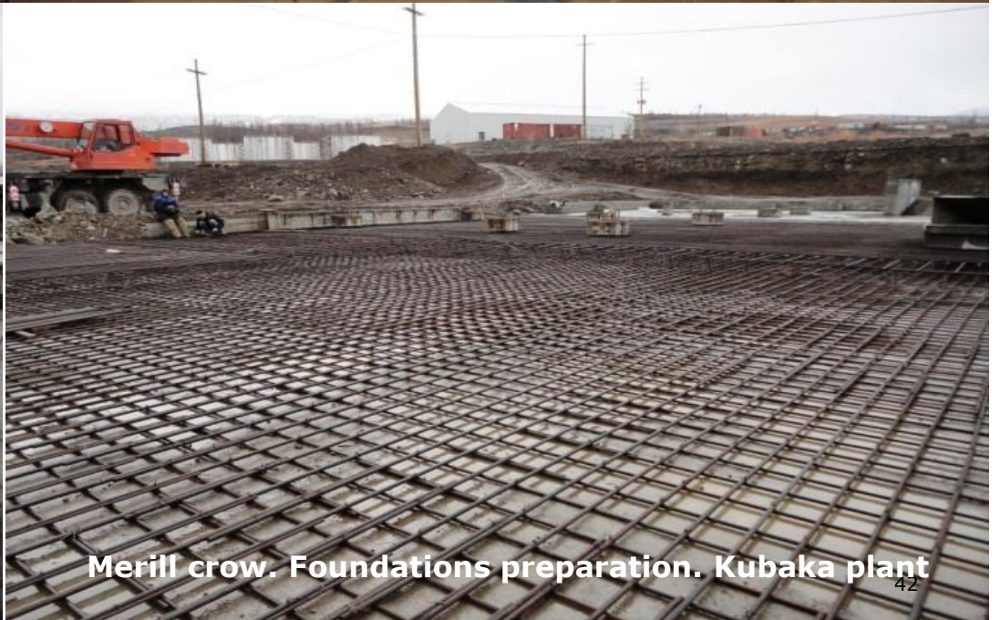
Construction of a new leaching circuit
