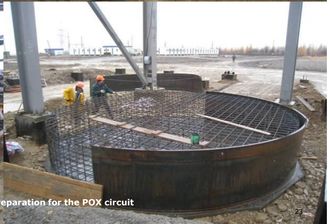
Structural steel framework for the POX plant
